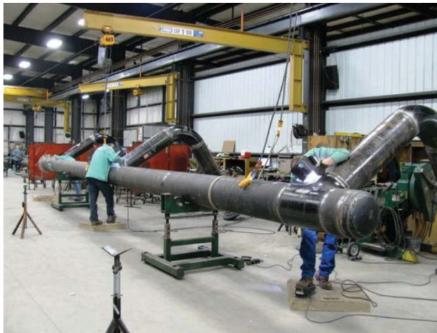
Gambar 1.4 Proses pengelasan pipa di bengkel. Sumber: Bohnart, 2018
