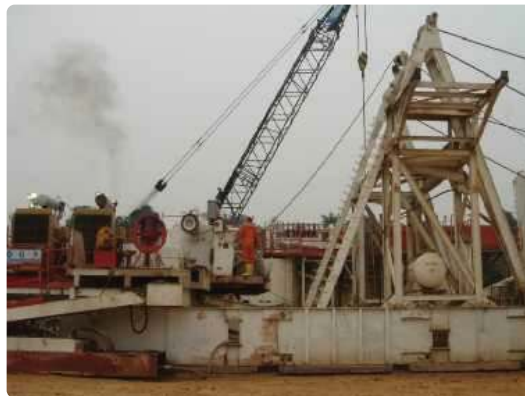
Gambar 6.6 Perangkaian Sub-structure Sumber: PPSDM Migas Cepu/Susilo (2012)
