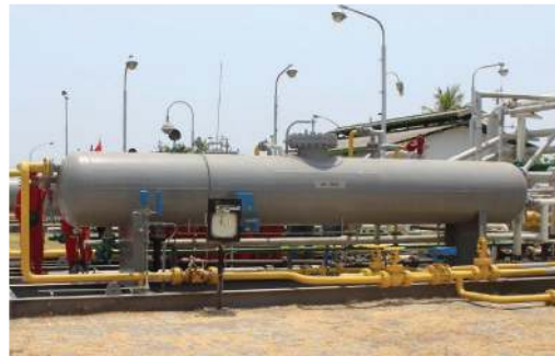
Gambar 7.26 Separator Horizontal Sumber: Yudanto (2013)
