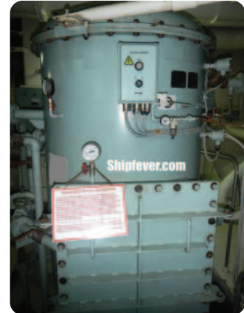
Gambar 9.24 Oil water separator Sumber: S.J. de Waard/en.wikipedia.org (2009)
