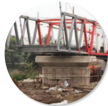
Gambar 6.17 Abutmen Jembatan
