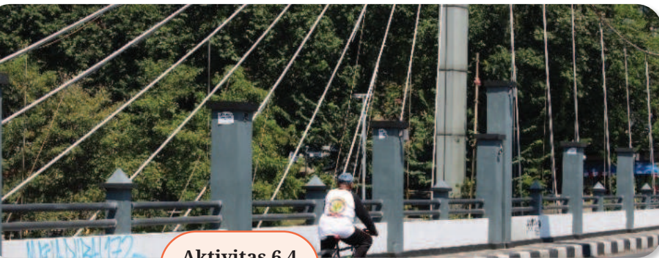
Gambar 6.19 Railing Jembatan
