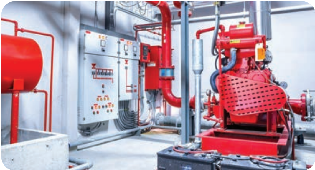
Gambar 2.16 Advanced Fire Detection (AFD)
