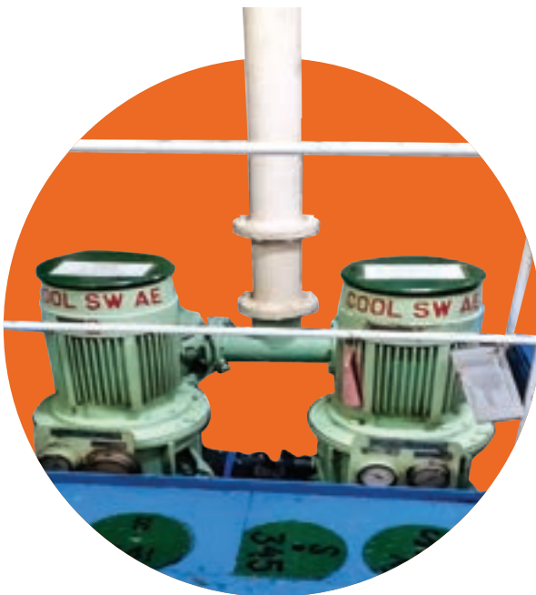
Gambar 2.8 Sistem Pendingin Air Sumber: Fino Waspodo (2024)
