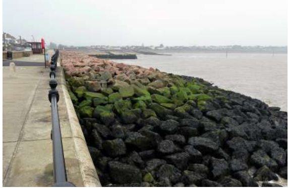
Contoh susunan batu revetmen Sumber gambar: Storye Book/CC BY 3.0
