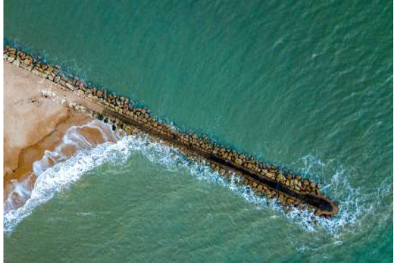
Contoh groynes. Sumber gambar: Ibu Suwaida Lahama, Ibu Mareeyoh Saemahsae, Ibu Isara Narawong, Ibu Rosakimi Hayee-arong, dan Ibu Aswaneer Mathawee
